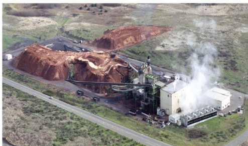
The Fairhaven biomass plant is an 18 MW generation facility located in northern California.
