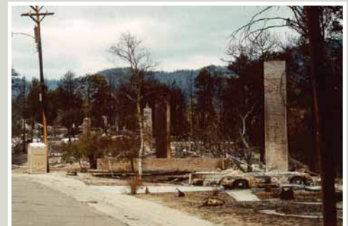
A structure destroyed during the Cerro Grande fire
